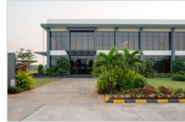
Laid foundation for Oncology OSD Plant in Visakhapatnam
